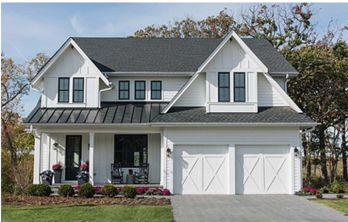
Garage not more than 55% of front façade, not set back more than 12 feet from primary façade
